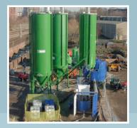
When S/S treatment is carried out *ex-situ* material is stockpiled and treated in batches using either an excavator with an Allu bucket attachment, a tractor pulled Stehr or a Wirtgen. Material is deposited in a sealed bunded area and the S/S additive(s) are introduced whilst the specialist plant combines them to form a homogenous mass.
