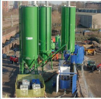
When S/S treatment is carried out *ex-situ* material is stockpiled and treated in batches using either an excavator with an Allu bucket attachment, a tractor pulled Stehr or a Wirtgen. Material is deposited in a sealed bunded area and the S/S additive(s) are introduced whilst the specialist plant combines them to form a homogenous mass.
